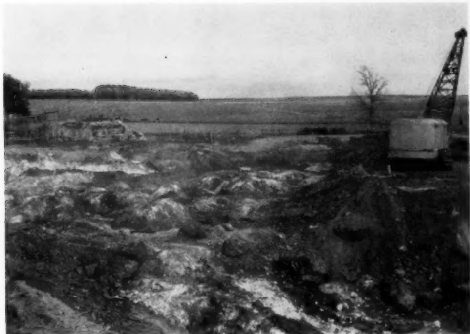
An iron ore pit showing the nature of the topography in the region of the iron deposits.
